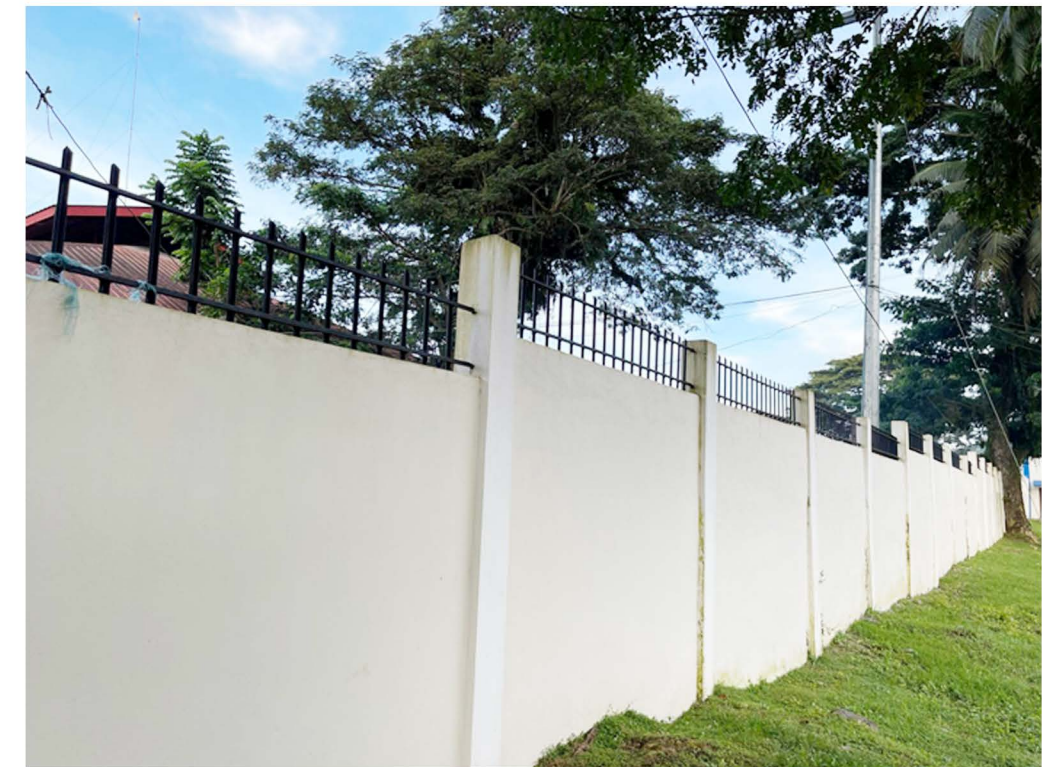
01 | Repair of Fencing - Main Campus
