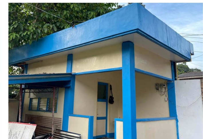
02 | Repair of Gate 1 and Guard House
